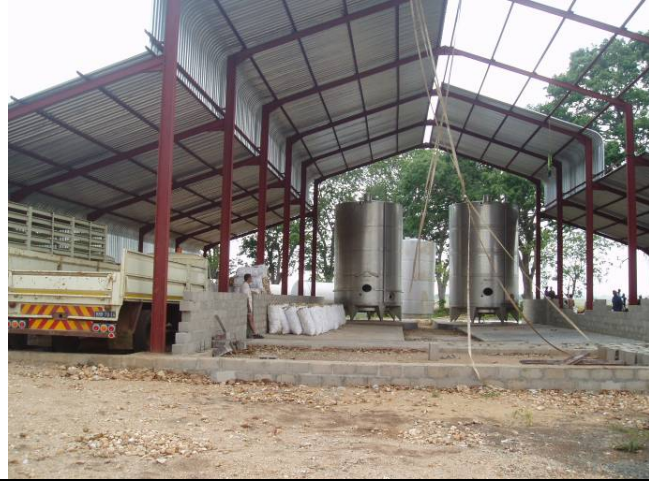
Figure 8. Ethanol Plant under Construction, Mocuba Mozambique
