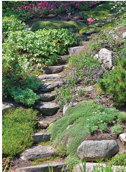
Rock steps with plants and gravel can absorb flowing water.
