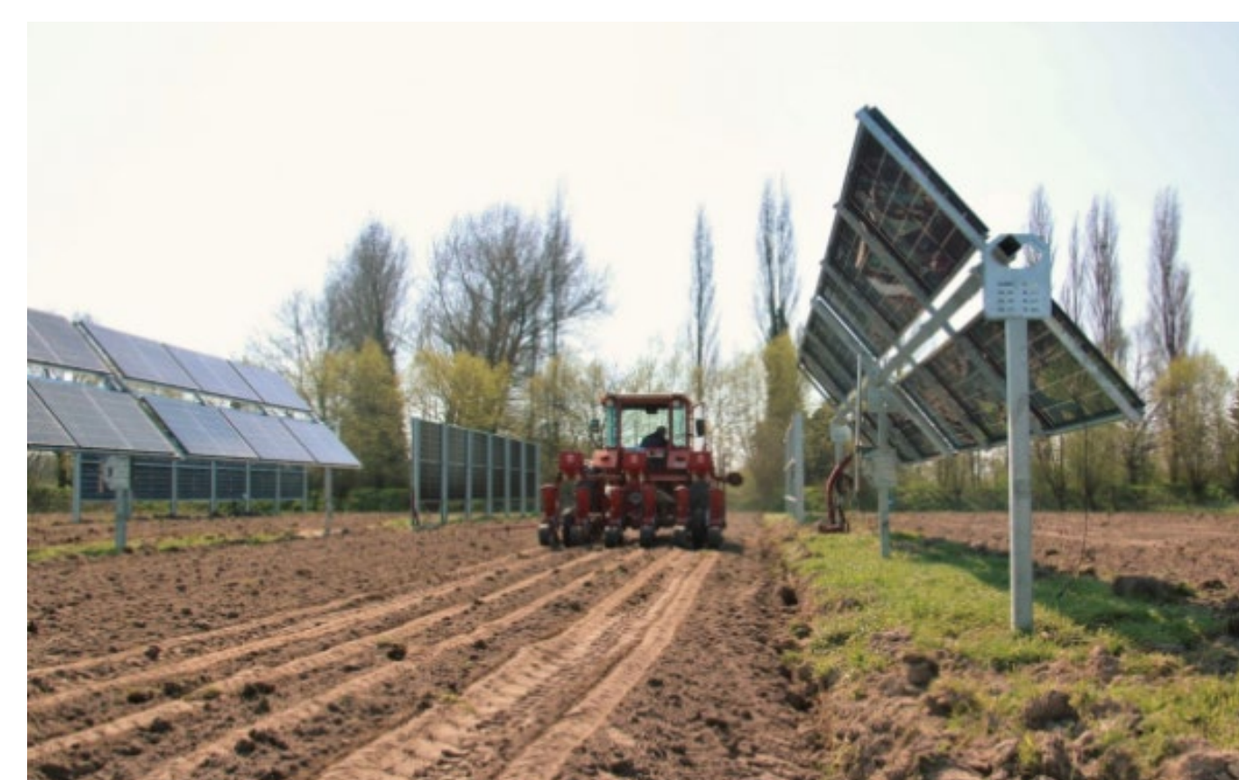
Figure 2. Example of a single axis tracking system in Grembergen, Belgium.
