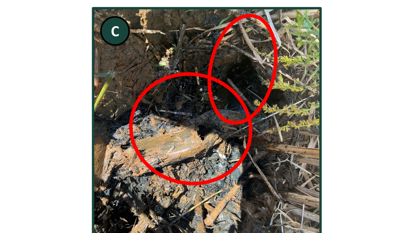
Figure 2 (A) Short-circuit pipe on side of Block A, (B) Manhole connecting Blocks A and B, (C) Broken Pipe covered in sediment and biomass
