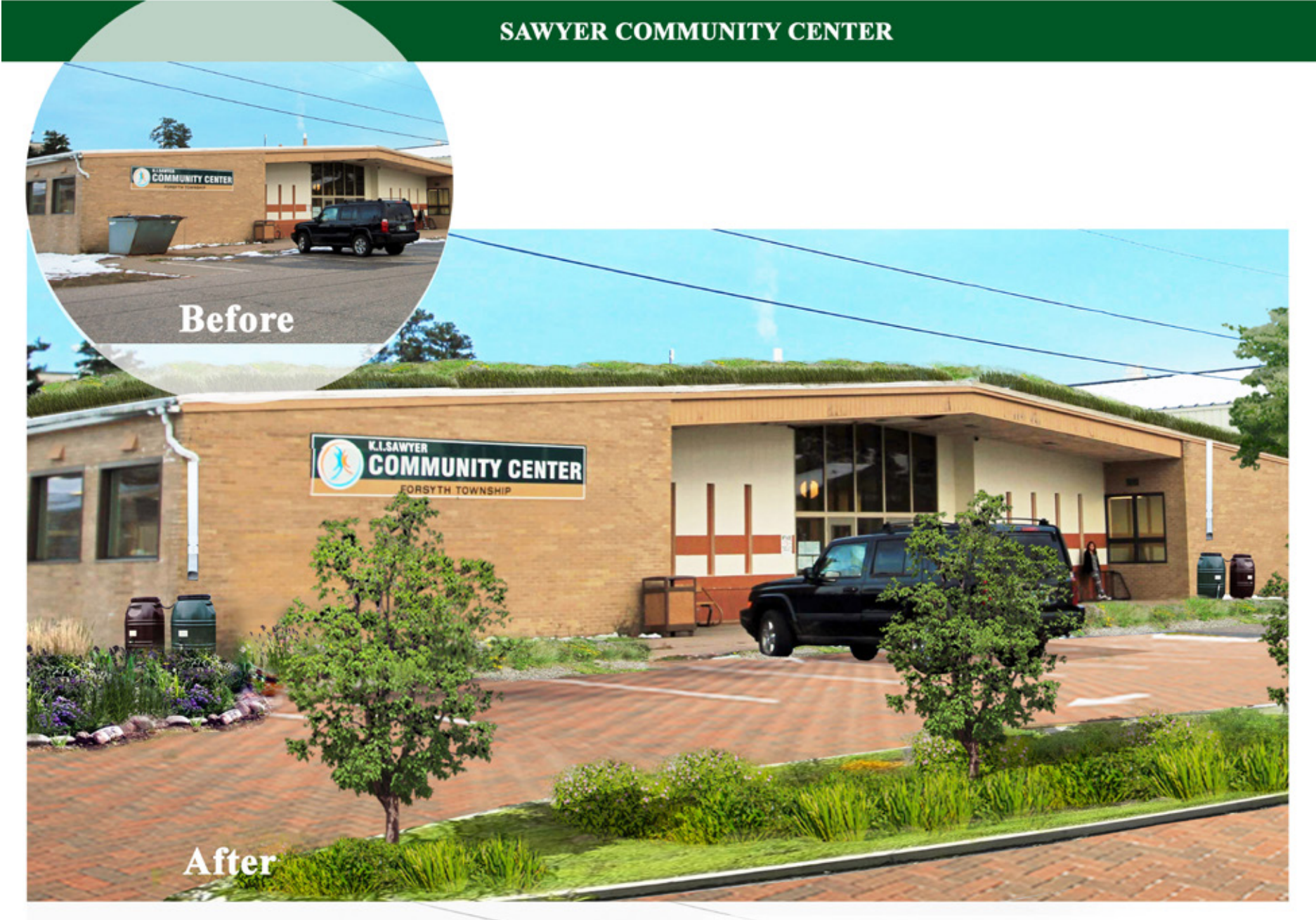
Figure 28a: Community Center in Marquette County before and after adaptation interventions.
