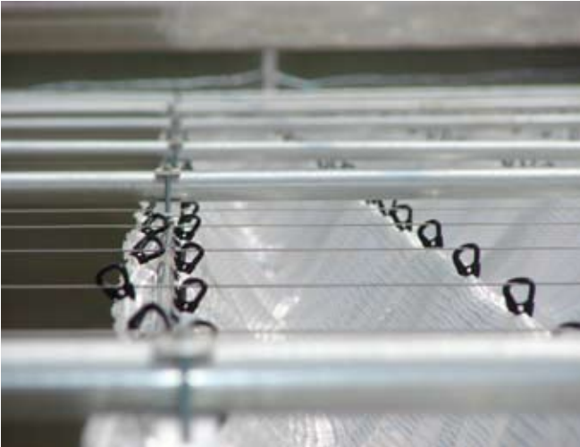
Top: Sliding installation.
