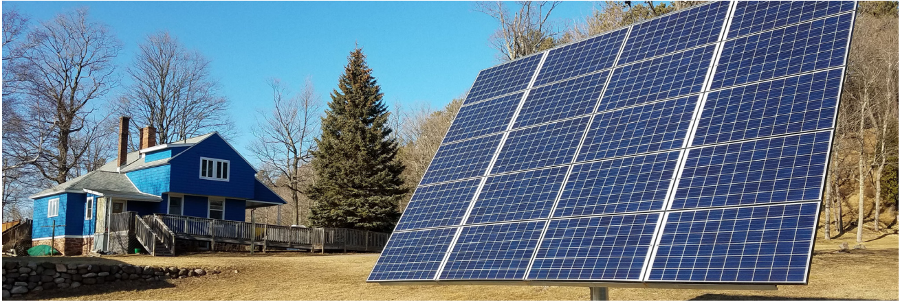
Ground-mounted monopole SES. Photo by Bradley Neumann.
