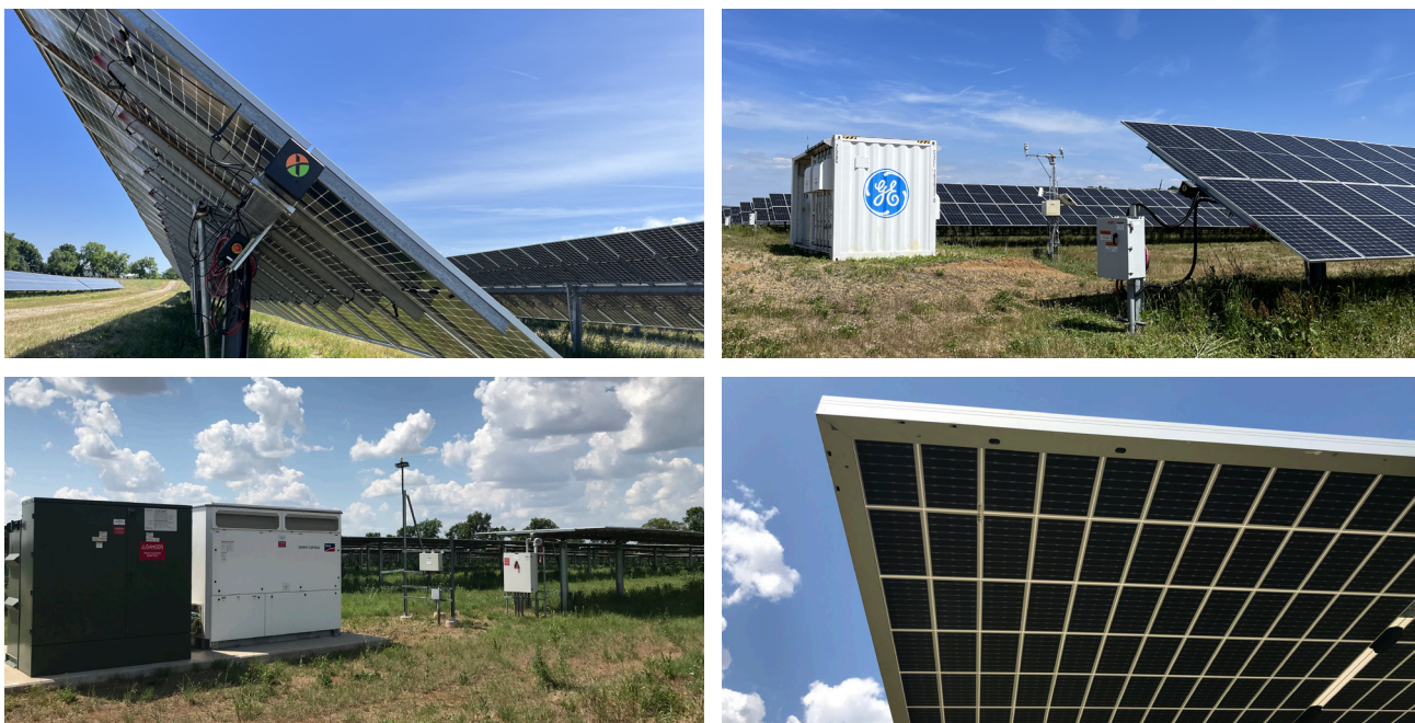
(Clockwise from top left) Racking and tracking system; inverter, weather station and collector box (both Madeleine Krol); bifacial panels; transformer and inverter (both Mary Reilly).
