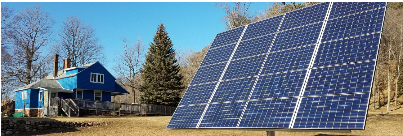
Ground-mounted monopole SES. Photo by Bradley Neumann.
