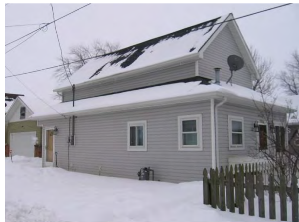
Figure 4.11 Housing in Block 3
