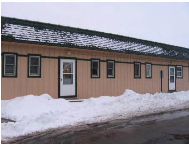
Figure 4.7: Vacant Building in Block
