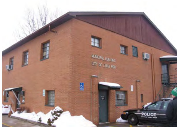
Figure 4.4: Luna Pier City Hall in Block 1
