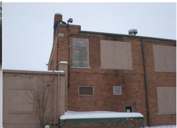
Figure 4.35: Vacant School Building
