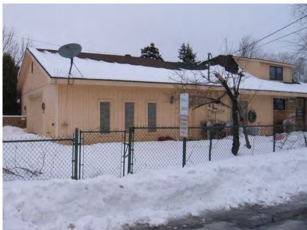
Figure 4.10 Housing in Block 3
