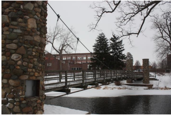
Figure 8: Bridge across the Shiawassee River
