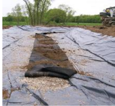
Figure 1: Filter strip lined bioretention channel under construction.
