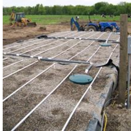
Figure 2: Constructed wetland nearing completion of installation.
