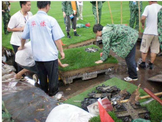
Image 4: China Sports Industry Group installing the final modules by hand at the National Stadium, Beijing, China, August 12, 2008, at 4:00 am.
