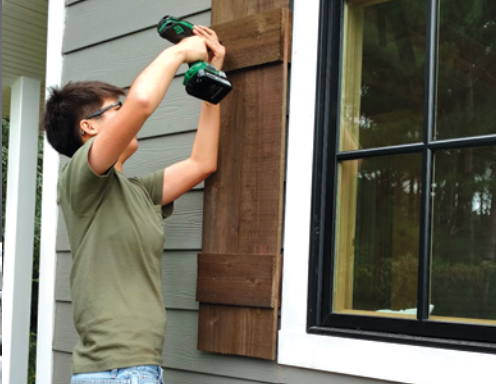
Hanbing Liang installing the shutters.
