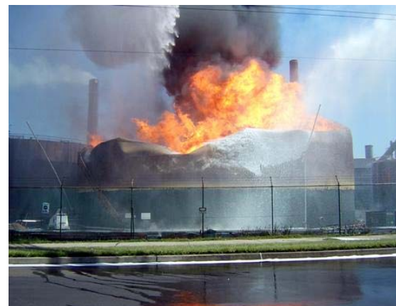
Ethanol tank explosion-- Tank roof blew off and fell on top of fire control systems rendering them inoperative
