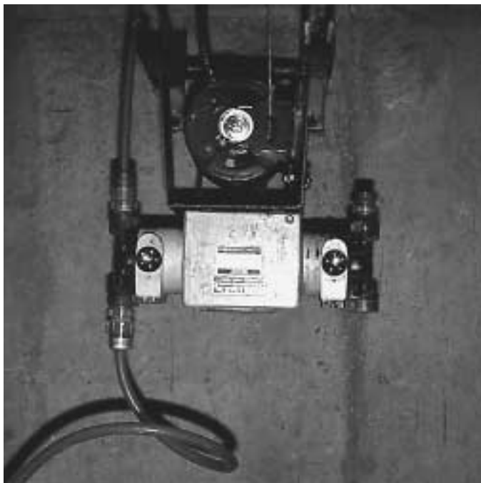
Chlorine-based chemicals must be fed continuously into the pool by an automatic or semi-automatic feeding system.
