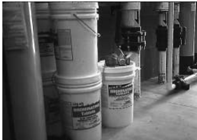
Store chemicals in their original containers in a cool, dry and secured location.
